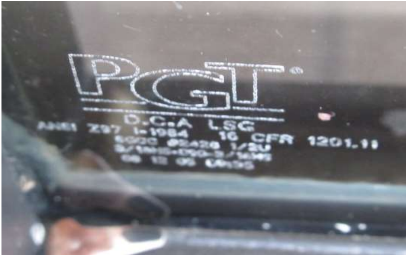
Slider glass etching (DCA LSG - Dade County Approved Laminated Safety Glass)
