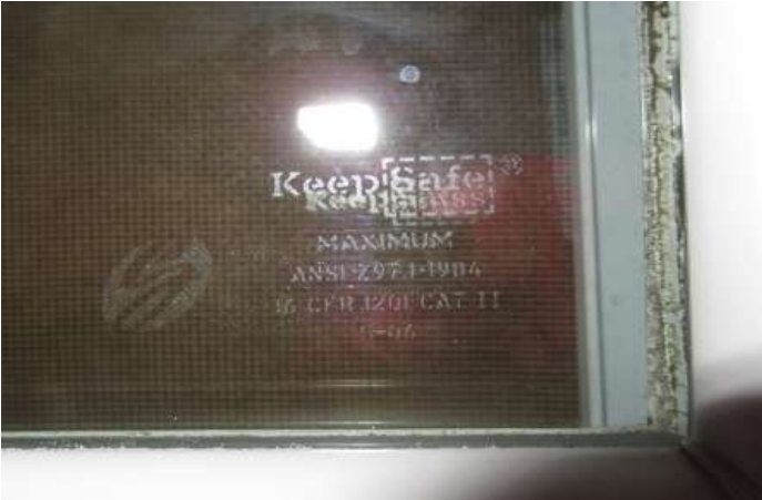
All stand-alone windows in the building meet the large missile impact standard (Keep Safe glass - maximum)
