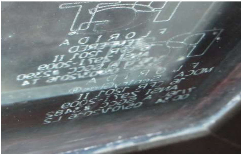
Slider etching (MDCA - Miami Dade County Approved)
