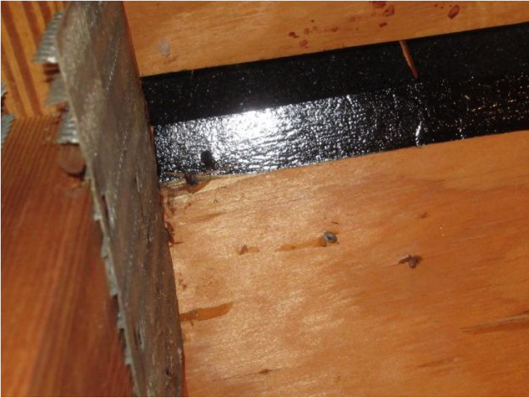
SWR installed under the metal panels
