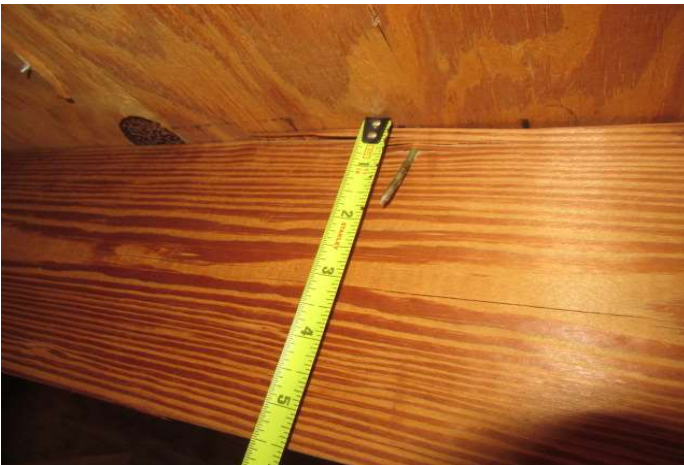
8d nails verified
