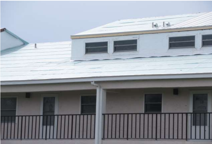
SWR installed under the metal panels
